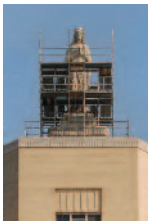
Top: guy-wires were wrapped around the statue to stabilize her. Left: scaffolding was erected less than 24 hours after the earthquake. Right: detail of some damage. Photos: Erik Highland/Superior Scaffold.
